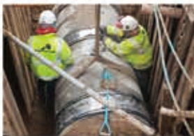
Large Dia. Pipe Replacement
