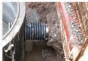
Connection of Existing Pipes
