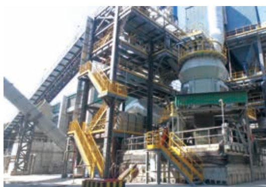
GGBS grinding facility in HK
