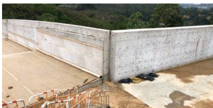
Retaining wall under construction using GGBS concrete
