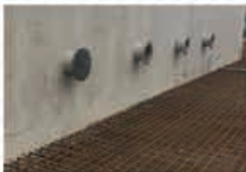
Water Cooling Tank
